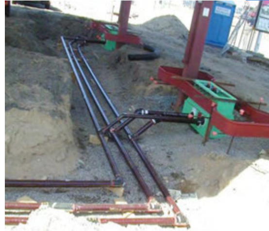
Figure 3.20: FRP piping during installation
