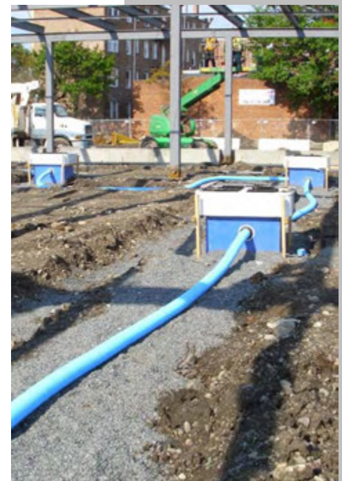
Figure 10.2: Underground piping connected to dispenser sumps before being buried
