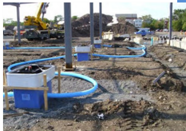
Figure 3.19: Flexible piping during installation
