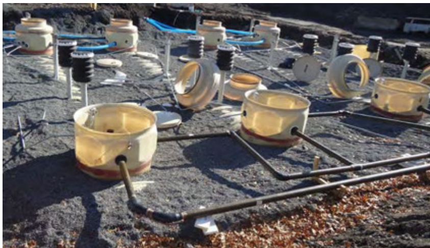
Figure 10.1: Underground piping system connected to tank top sumps before being buried
