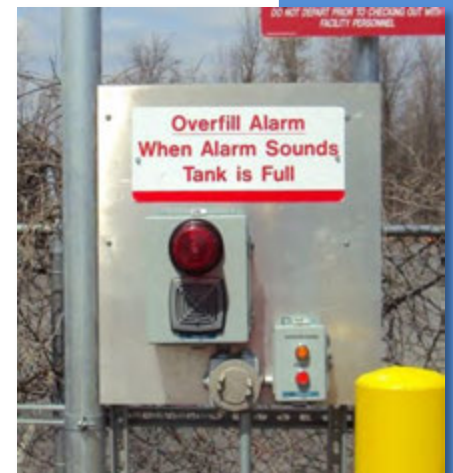
Figure 7.5: Electronic overfill alarm
