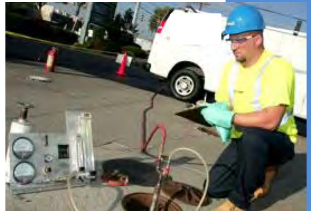
Figure 14.7: Technician performing a tank test
