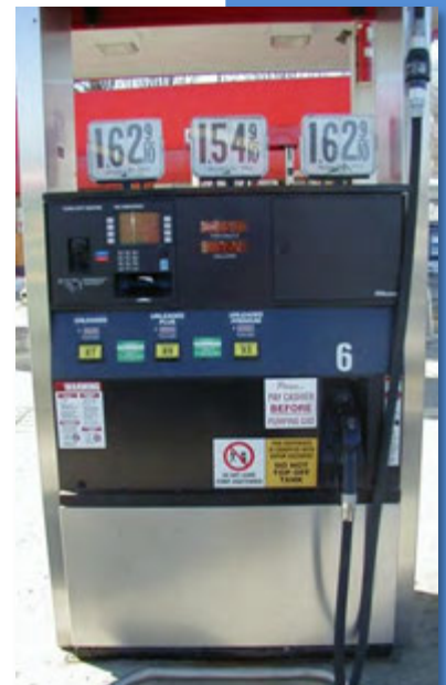
Figure 12.7: Typical retail dispenser with blending to dispense 3 grades of fuel
