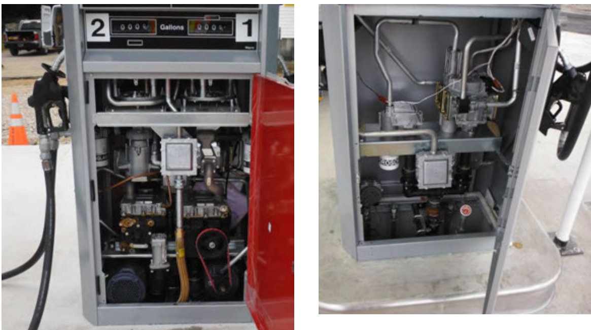
Figure 3.15: Suction system dispenser (left) and pressurized system dispenser (right).
