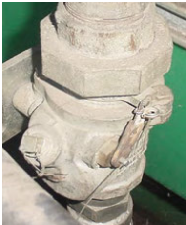
Figure 12.11: Retrofitted shear valve. This defeats the safety purpose of the valve and would fail a DEC inspection.
