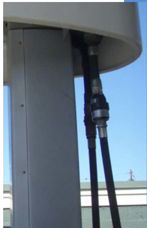
Figure 12.17: Breakaway valve
