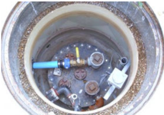
Figure 3.13: Suction piping system
