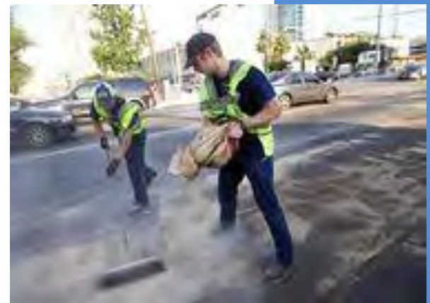
Figure 18.5: Workers put spill absorbent on a spill. Should your Class C Operators know how to use absorbent in a spill situation?
