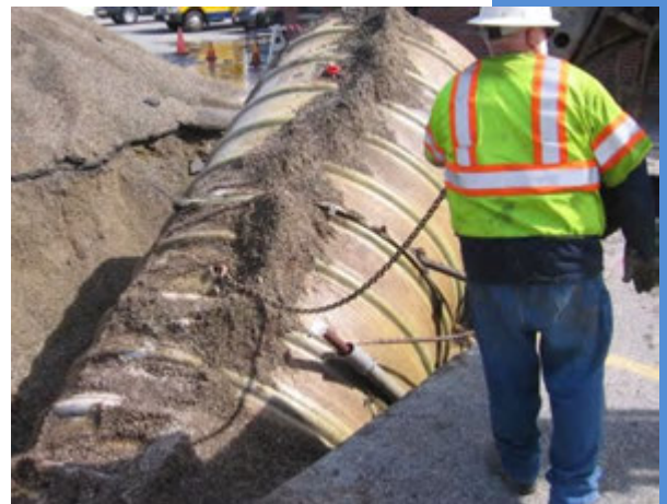
Figure 6.2: Tank Removal
