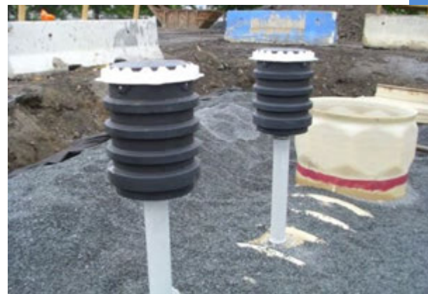
Figure 3.17: Spill bucket
