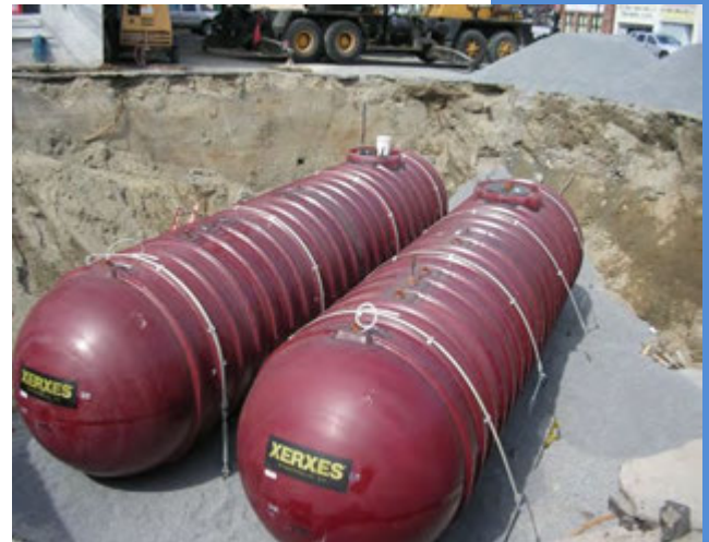
Figure 3.4: Double-walled FRP tank ready for installation
