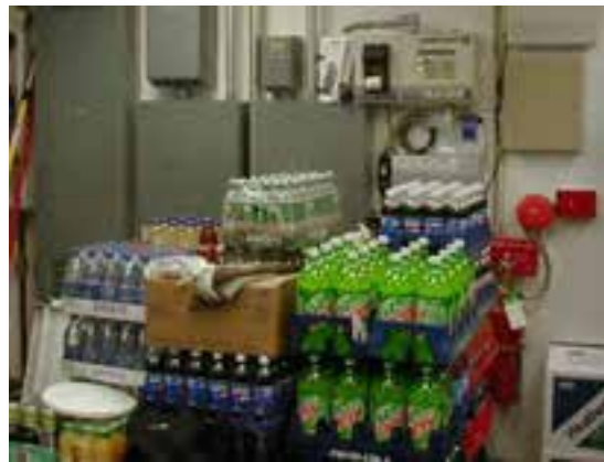
Figure 9.7: ATG console that is not accessible
