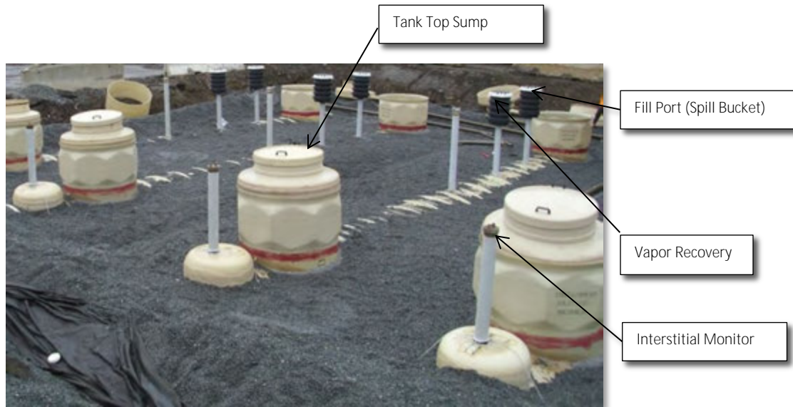
Figure 3.10: Common service station UST layout
