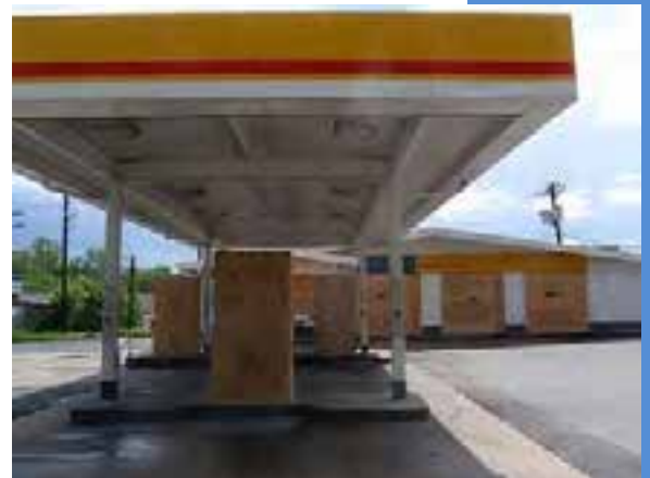
Figure 6.3: Out-of-service tank systems must be maintained until permanent closure.
