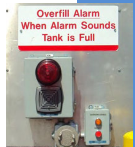
Figure 3.26: Overfill alarm
