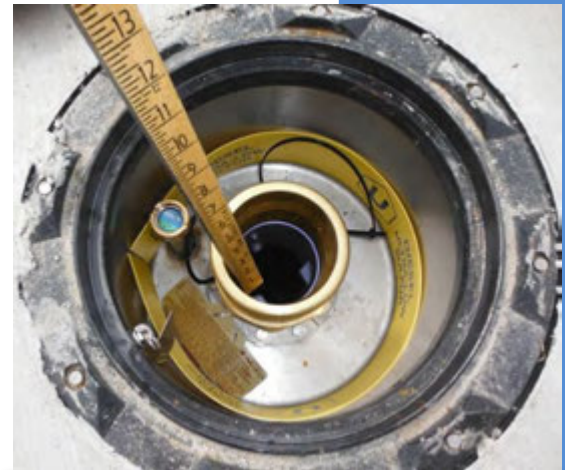
Figure 8.2: Measuring tank level with gauging stick
