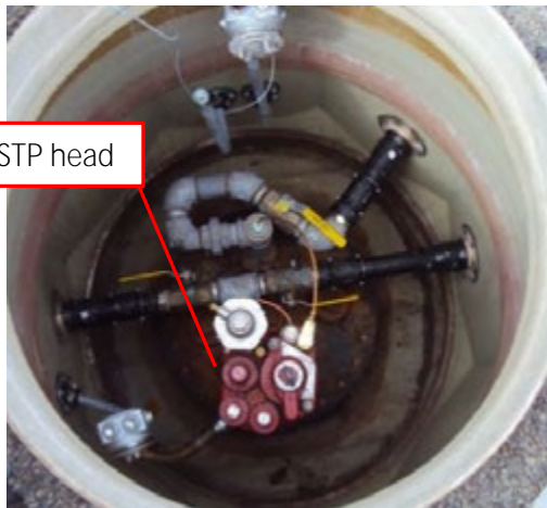
Figure 10.3: Pressurized pumping system
