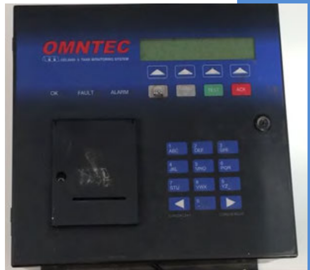
Figure 8.1: ATG system console (example of one make/model)
