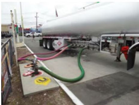
Figure 13.1: Fill hose connected to fill port inside a spill
