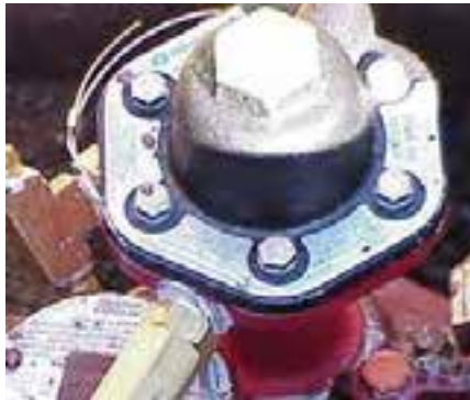
Figure 10.5: Mechanical LLD (Alaska DEC)
