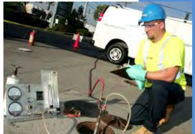
Figure 9.12: Technician performing a tank test
