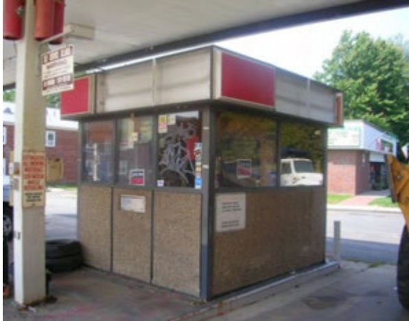
Figure 6.1: Out-of-Service Gas Station
