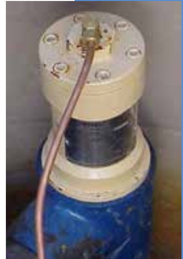
Figure 10.6: Mechanical LLD (Alaska DEC)
