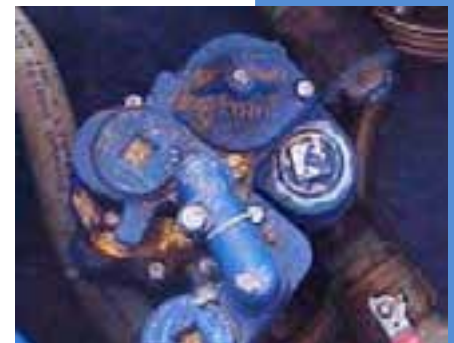
Figure 10.8: Submersible pump with no LLD
