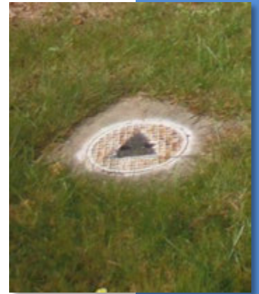
Figure 3.24: Monitoring well
