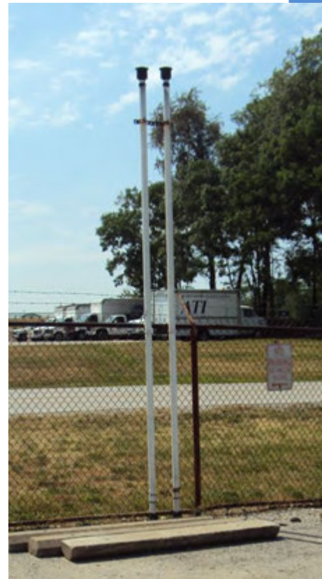
Figure 3.21: Vent stack arrangement
