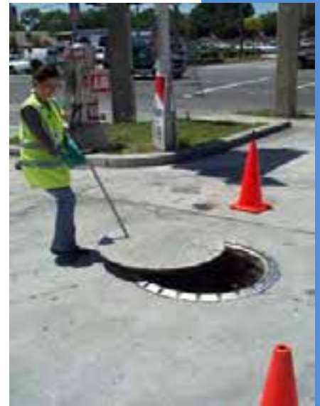
Figure 2.1: Operator opening a tank top sump. Class A and B operators are responsible for tank maintenance and monitoring
