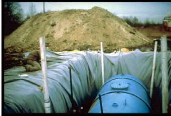
Figure 9.4: Tanks being installed with a secondary barrier
